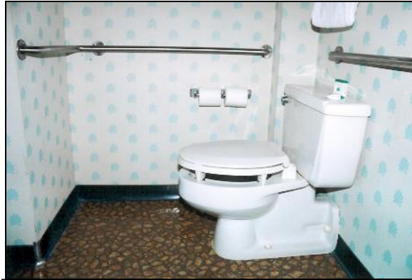
Accessible bathroom with grab bars, properly positioned toilet paper holder and toilet seat with risers.
