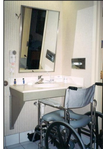
Tilt mirror, lever water control, sink roll-in height 29 inches, & the pipes are covered.
